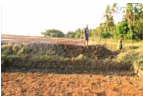
Photo2: Embankments in Auk Seik Kwin village
