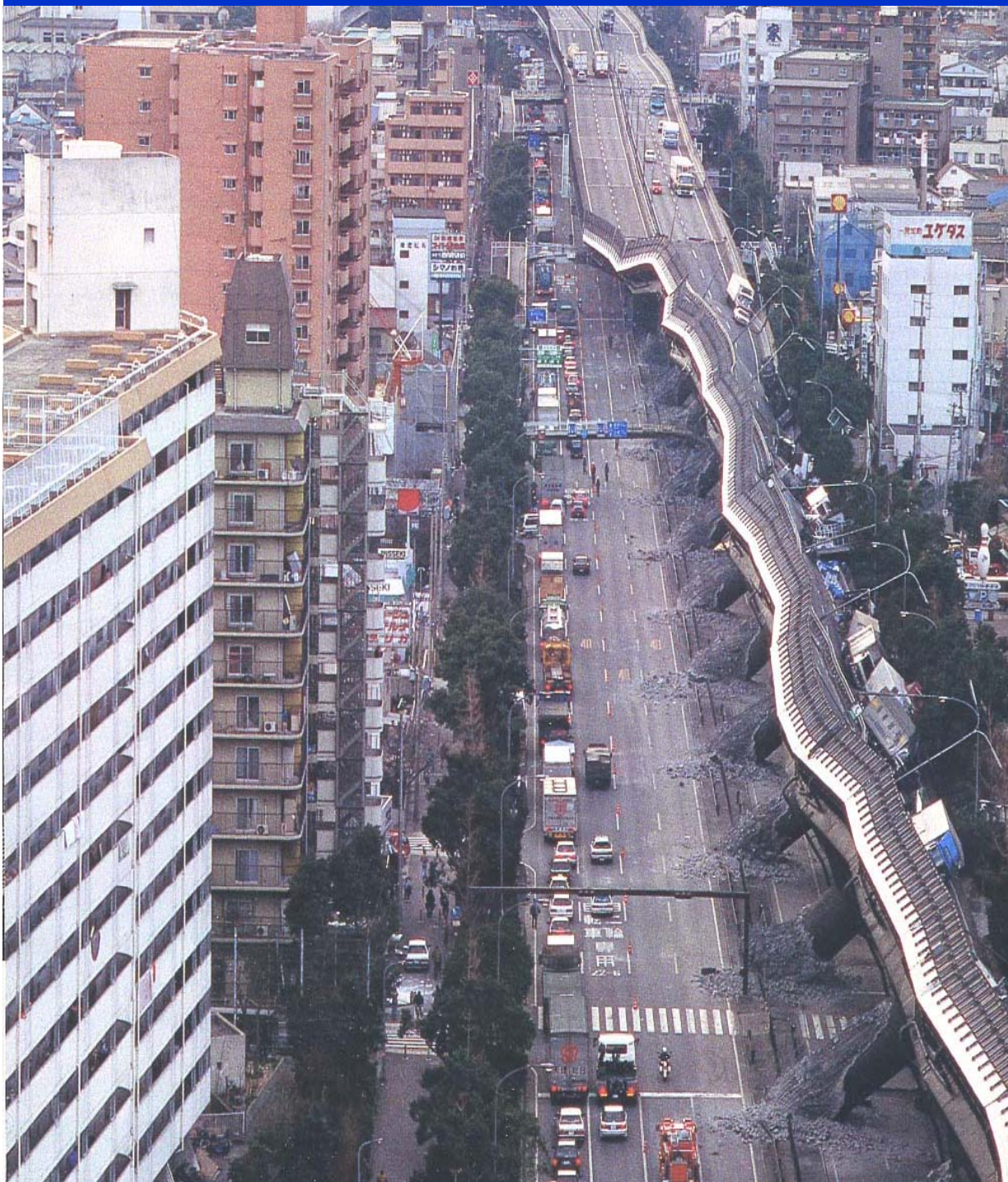
Shear failure of large bridge piers in Kobe Earthquake, 1995
